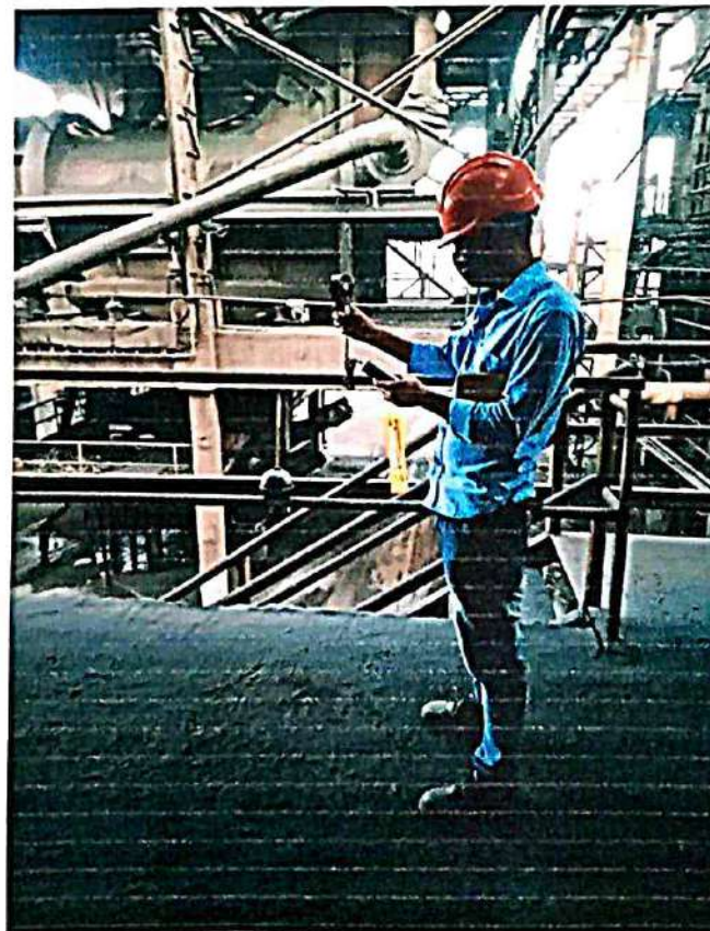
DRI 3 DSC AREA
