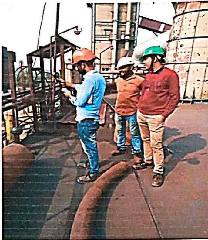
Pellet 1 Cooler Floor Photo
