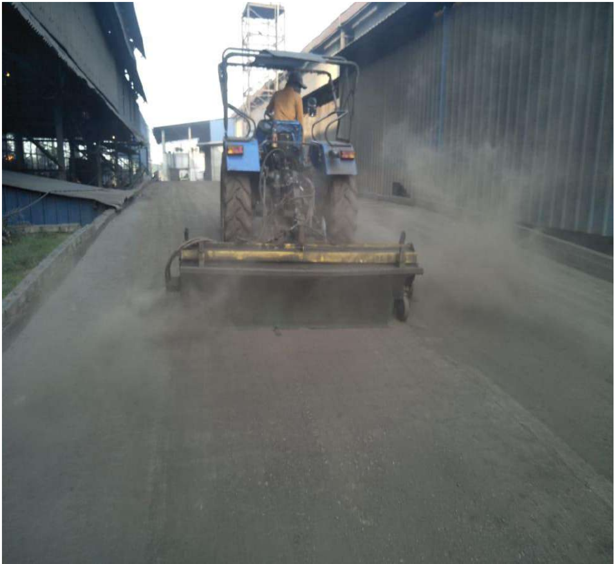
MECHANICAL SWIPING MACHINE AT WORK ON THE ROAD
