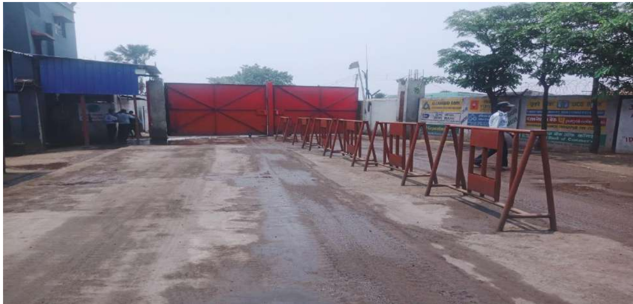
RCC ROAD STARTED INSIDE FROM MAIN GATE OF THE COMPANY
