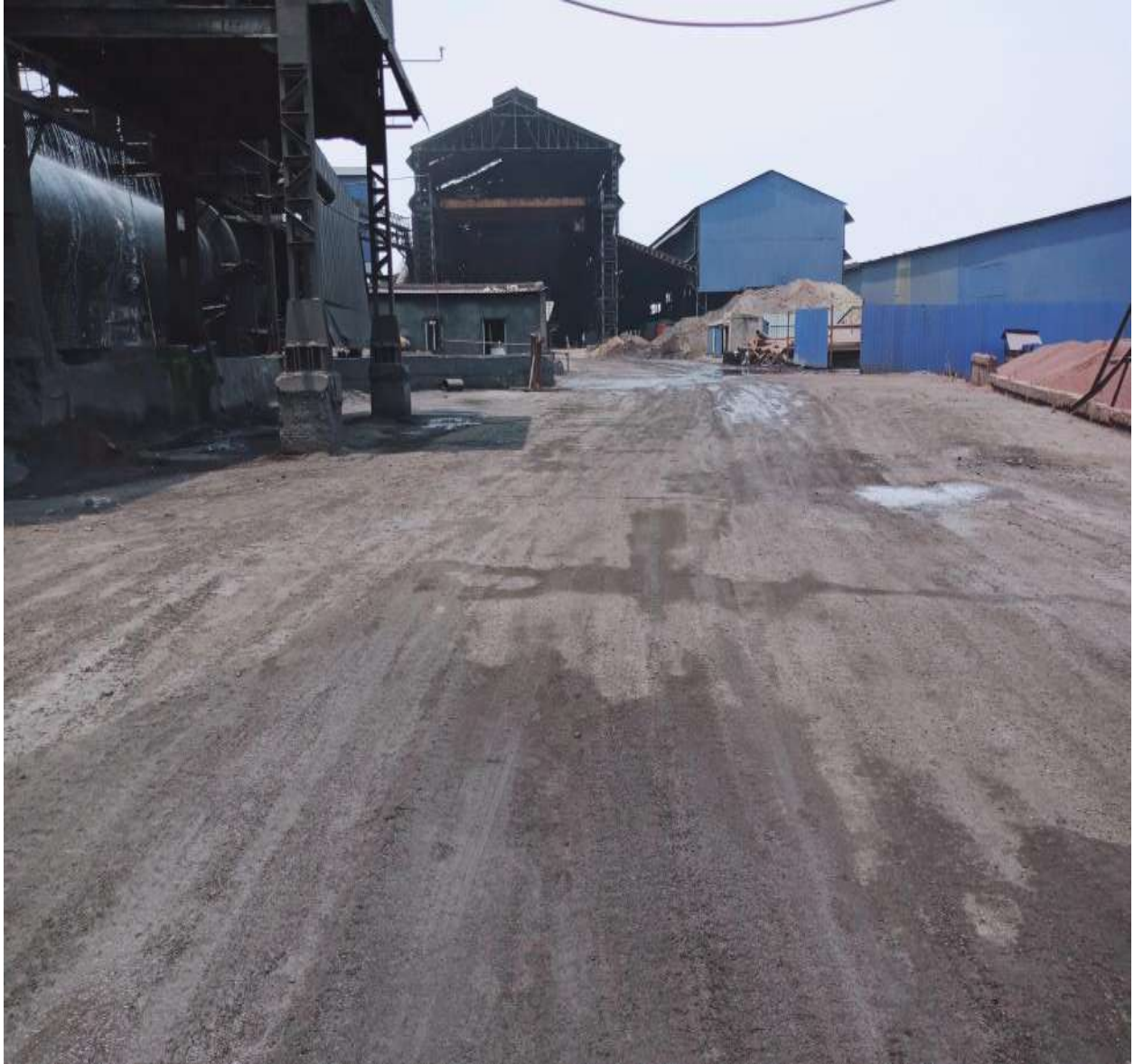
RCC ROAD INSIDE THE FACTORY ALONG WITH WATER SPRINKLING
