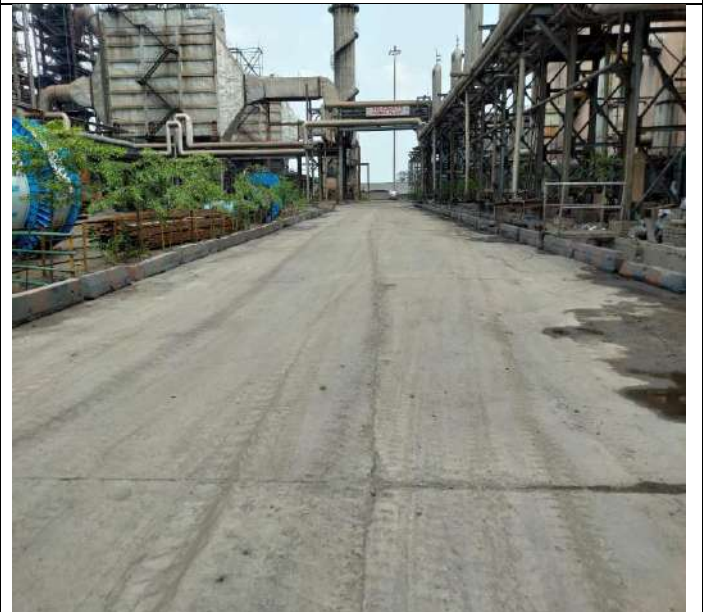
RCC ROAD AND PAVER BLOCKING IN THE PLANT AREA
